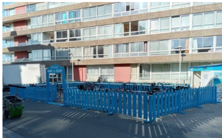
Figure 16 : Fence for a bicycle park made from non-returnable pallet wood
